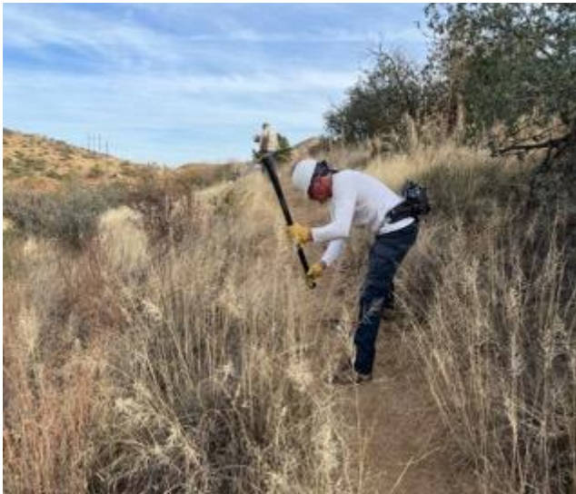
Catclaw roots are dug out to prevent regrowth on the trail. Photo by Elisabeth Wheeler
