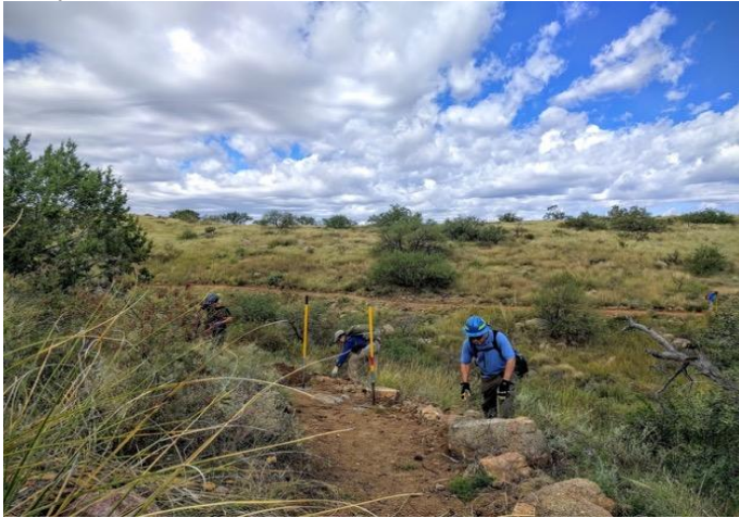
Brenda Dawson and Roddy Wilder are working on drainage issues.
